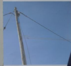
Illegal connections are carried by attaching the wires to existing telephone or electricity poles.
